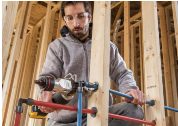
EVERLOC+ Residential Installation-1 EVERLOC+ ® compression-sleeve fitting system in 1/2-inch diameter in residential plumbing application ©REHAU
